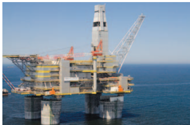
Lunskeye A: a concrete gravity base structure at Sakhalin II.
