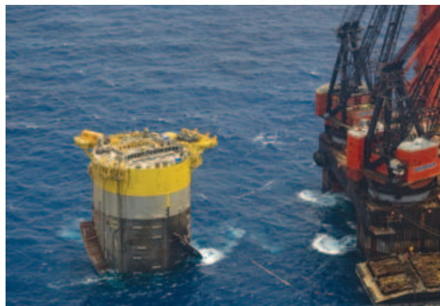
Shell's Perdido spar being installed in the Gulf of Mexico, August 2008.
