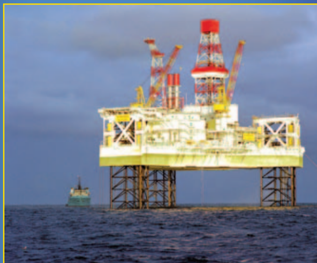
Harding platform is an example of how long-term recovery processes can be optimised through the use of emerging technologies. Photo credit BP
