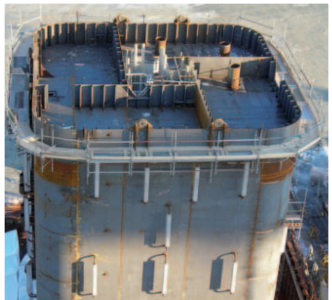
Blind Faith hull under construction
