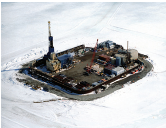
Drilling operations in remote areas rely on first-class logistical support.
