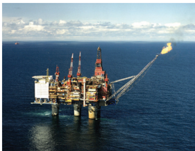
Several fields have been connected via tieback to the Gullfaks C platform.
